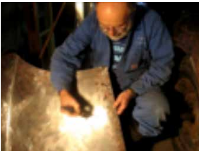
Figure 1 - Numerous rust holes in the outer skin
